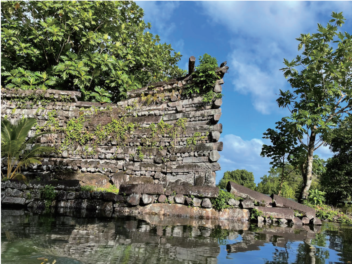
Figure 1. Nan Dowas at Nan Madol displaying the columnar basalt from which it was constructed.
